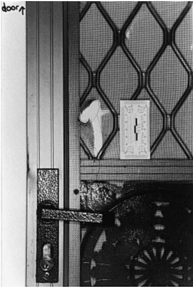
FIG. 1—Damage to security door—inner face.
